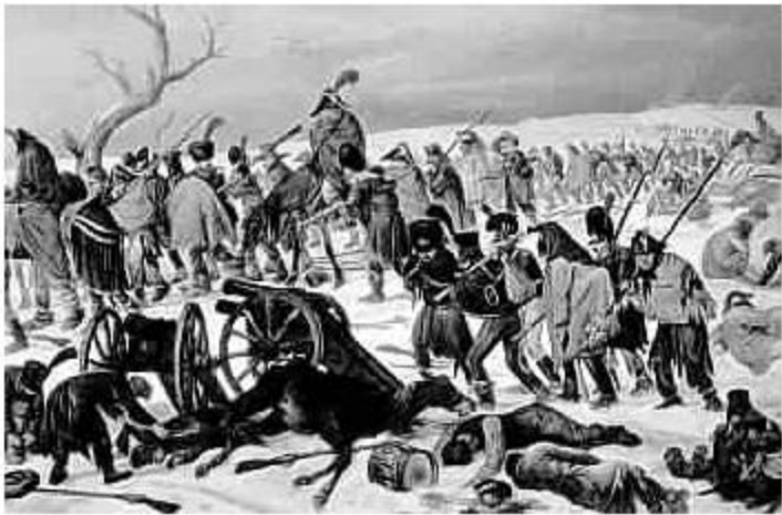
Napoleon's Failed Invasion of Russia – 1812 *
